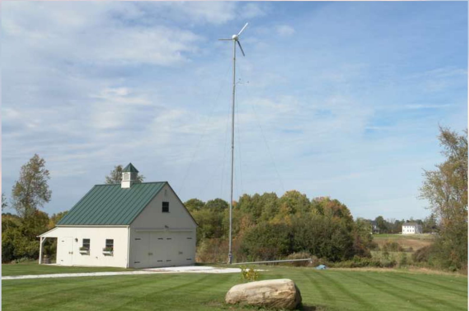
2.5 kw ET turbine in Shelburne, VT
