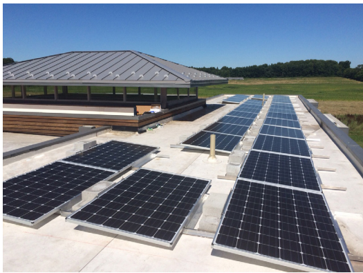
30 285 W SolarWorld modules Fronius Primo 7.6 kW inverter, 8.55 kW DC
